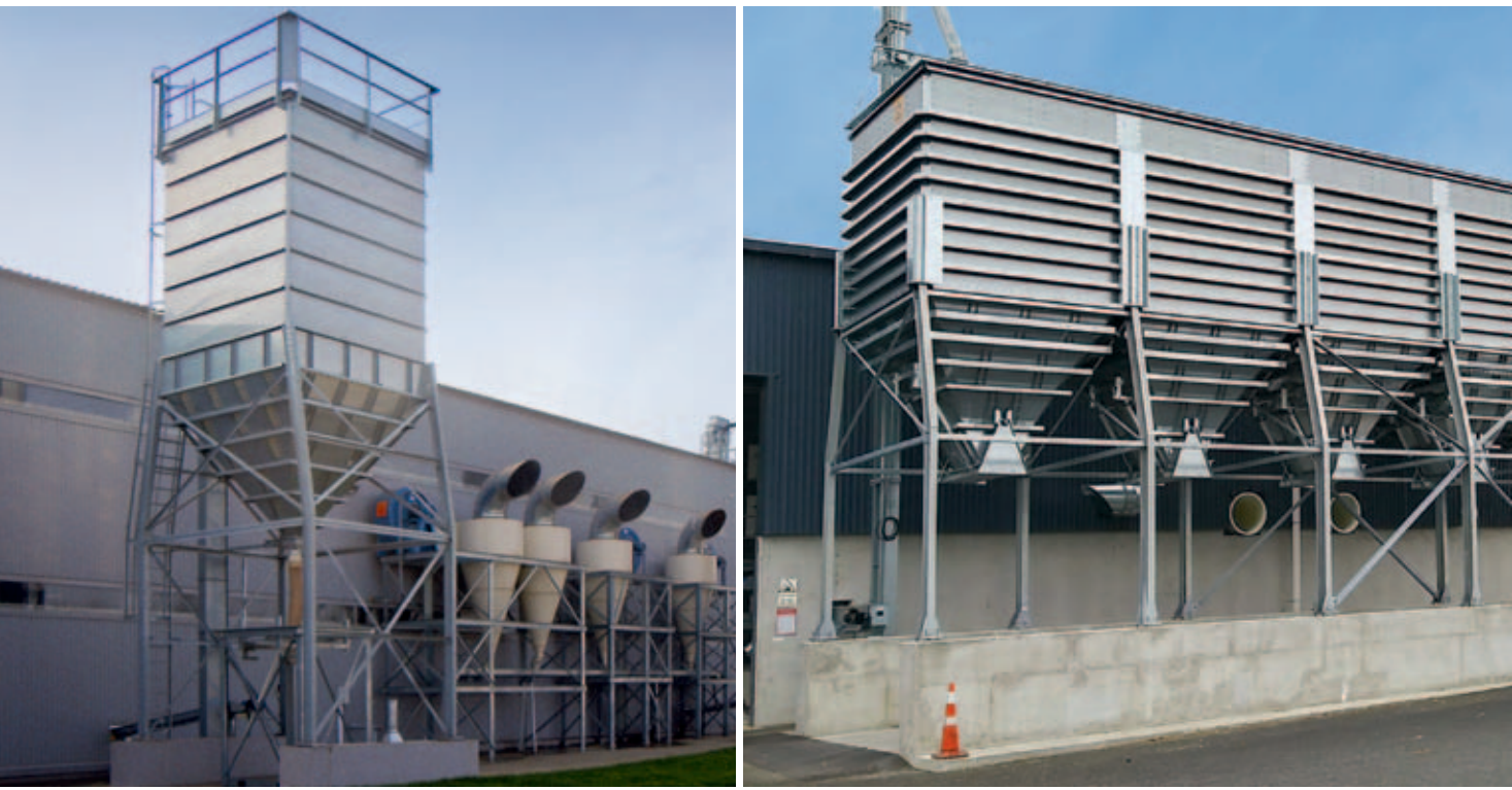
Buffer with tension bracing for waste and grain
