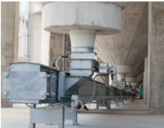
Flat-bottom silo FBS with concrete hopper
