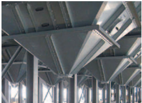
Hopper 45° in segment design
